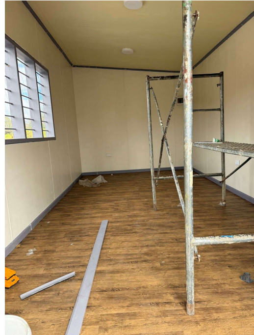
Left: staging materials and equipment on site, with both completed buildings visible in the background. Right: interior fit-out work underway inside one of the new buildings.
